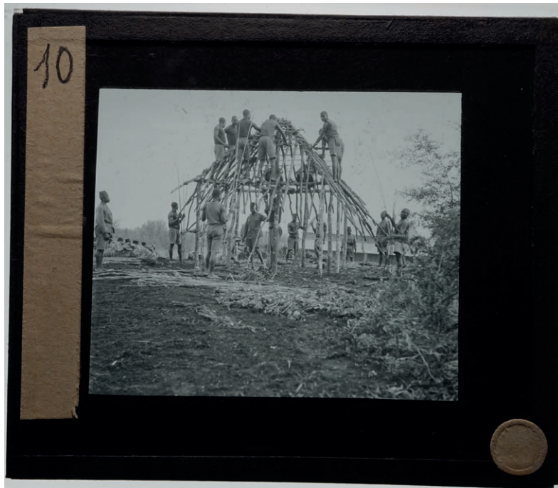
Figure 12. Construction of a meteorological observatory in Beni. "The observatory is built in matt. This type of house costs just a few francs."
