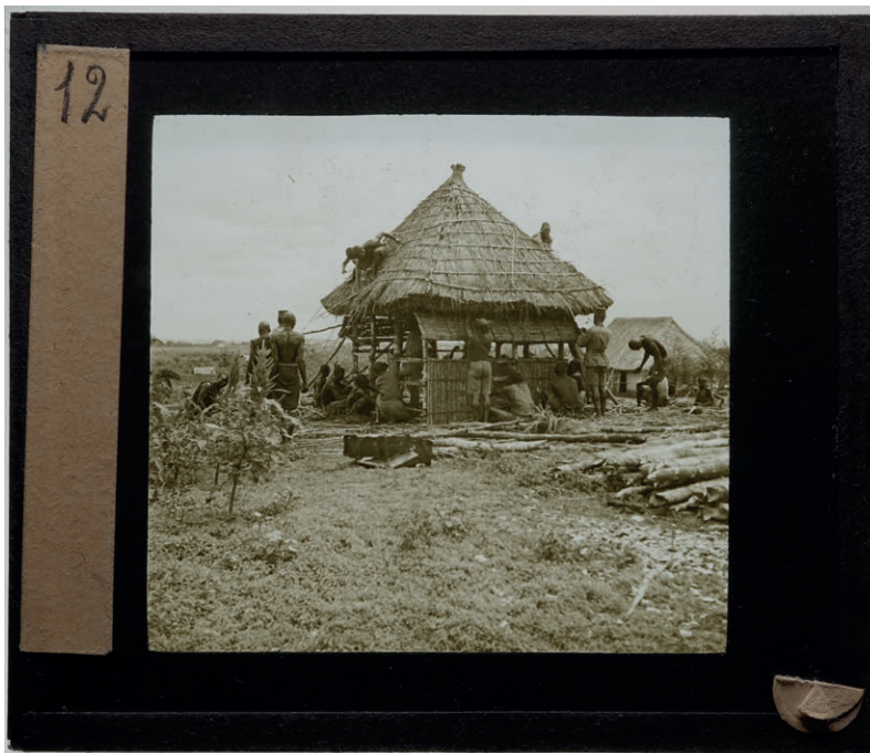
Figure 13. "The observatory is almost complete. Throughout the mission, all the meteorological observation data will be regularly recorded, as will be done at all the camps."
